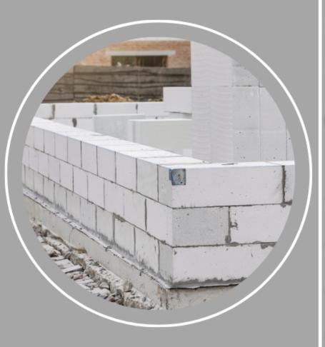
essential role in a variety industries, including civil engineering, by providing answers to issues such as global warming and raw material scarcity. In order to meet demand Autoclaved aerated concrete (AAC) blocks are made from the above-mentioned raw ingredients, as well as some additional inert elements,...
