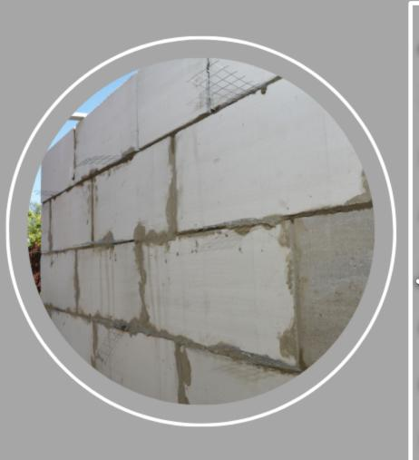
Autoclaved Aerated Concrete (AAC) is a lightweight aggregate masonry building material which can be used as infill, as sound control in walls, and as slabs for floors. AAC Blocks from A autoclaved aerated concrete (AAC) is a lightweight aggregate masonry building material which can be used as infill, as sound control in walls, and as slabs for floors.
