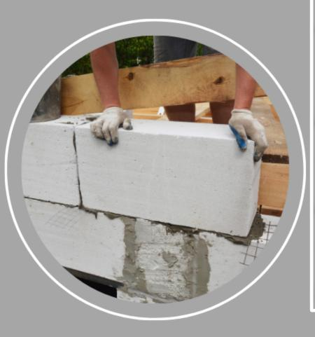
AAC Blocks are made of silica sand and lime stone powder and cement. It's produced by Autoclave process. The blocks excellent thermal insulation properties. They also have high abrasion resistance, with an impact strength like granite.
