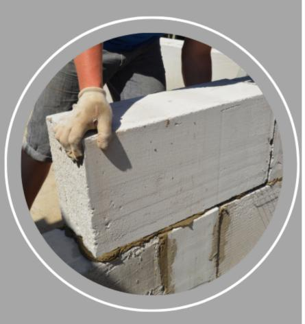
The product's ability to withstand water damage makes it ideal for both residential commercial applications and like driveways, patios and sidewalks. It can also be used as an insulator; if you live in an area where temperatures drop below freezing during winter months, using AAC blocks between your home and exterior walls can save energy costs.
