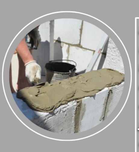
building materials lose strength when they're exposed to water, but autoclaved aerated concrete blocks are durable enough to be used in areas that are prone to flooding. If a hurricane or flood is on its way, adding AAC blocks in affected areas can reduce damage.
